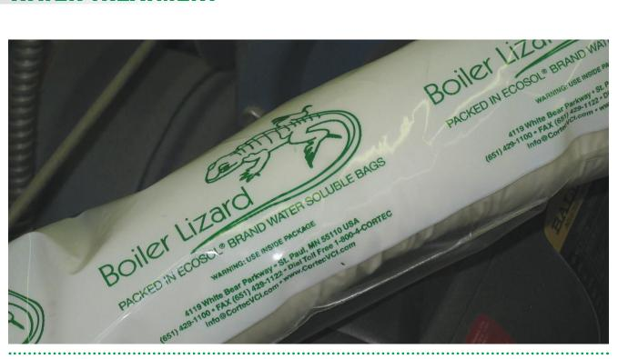
A vapor corrosion inhibitor packaged in a water-soluble pouch provides dry internal protection to boilers. Such materials typically can be left to dissolve inside the boiler when it is refilled.
