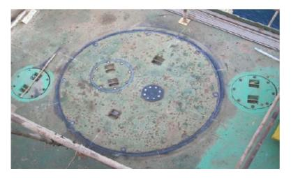
Figure 5: Caisson Leg Sealed Cover
