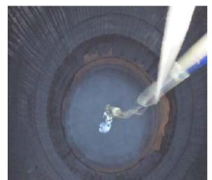
Figure 2: Application of Inhibitor A using a pipe coater
