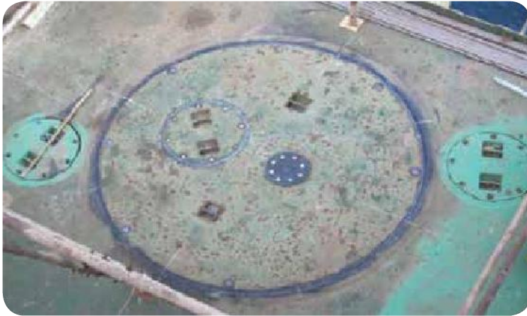
FIGURE 5 Caisson leg sealed cover.
