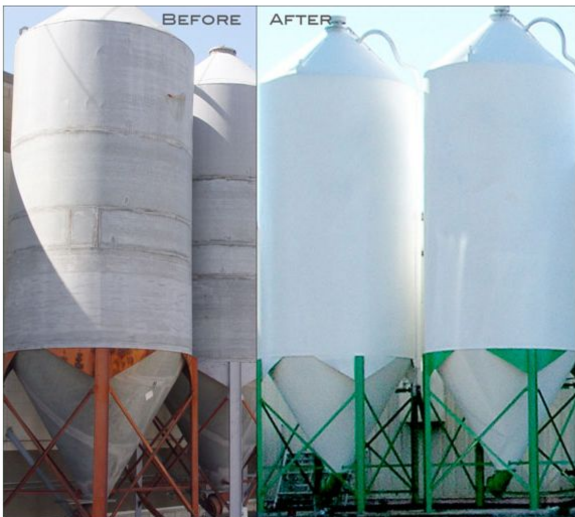
VpCI® 386 White, applied over weathered galvanized steel offering 10 + years of corrosion protection.
