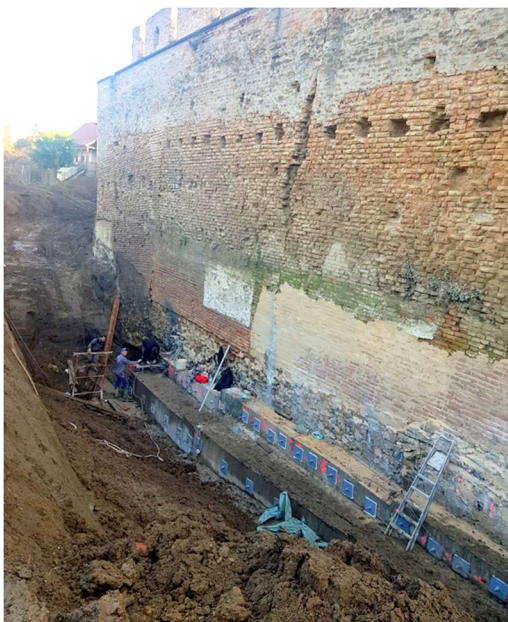
Reinforcement of the foundation of medieval city walls with MCI® Technology.
