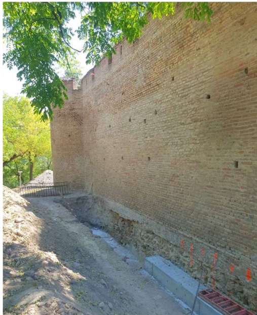
Reinforcement of the foundation of medieval city walls with MCI® Technology.
