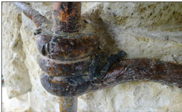
Damaged Joint
