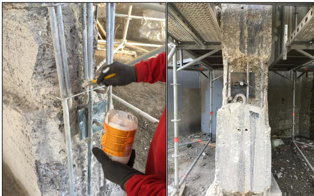
After rust and scale have been mechanically removed, CorrVerter MCI® was applied to heavily corroded metal surfaces of the water tower. They have been unprotected and rusting for over 20 years since the war ended.
