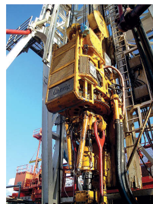
Outer surfaces of an offshore platform top drive unit were washed with VpCI cleaner/degreaser and coated with a VpCI outdoor corrosion inhibitor before temporary storage on deck for one year (source: Cortec Case History 303)
