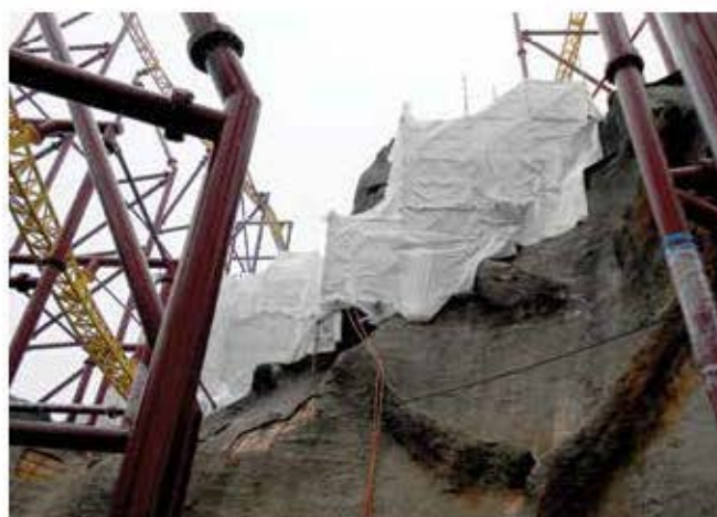
Fig. 12: Scaffold and the plastic protection over the mountain areas to be repaired Photo by Ray Schallom
