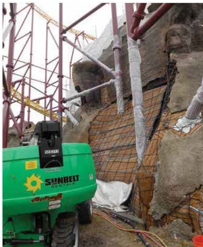
Fig. 9: The 0.375 in. (9.5 mm) V-shape lath, the rubber boot around the pipe support, and reinforcement to be encased into the silica-fume shotcrete Photo by Ray Schallom
