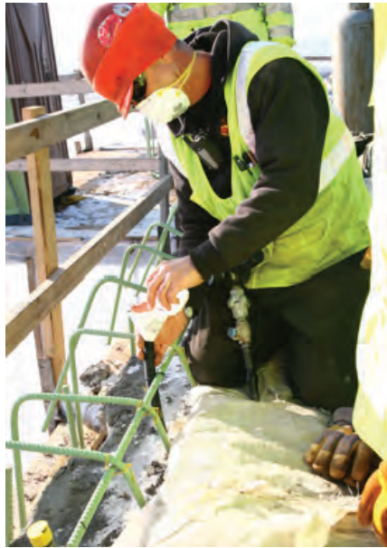
MCI-309 is easy to apply to PT ducts and does not need to be flushed out before grouting.
