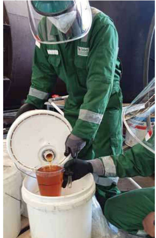
➤ Measuring Corrosion Inhibitor for Hydrotesting. Image courtesy of Tiga Ombak, Cortec® Case History 852.
