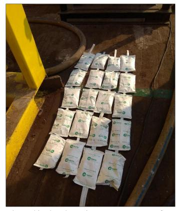
the piping. This film inhibits corrosion on the metal it is directly touching but also emits vapors to protect surfaces in harder to reach areas that may have been missed during application.
