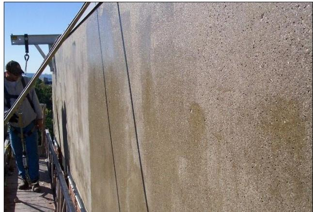
\* Surface Application Corrosion Inhibitor
