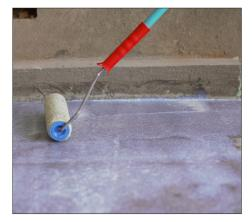
We are pleased to introduce our new surface prep guide for MCI<sup>®</sup> surface applied corrosion inhibitors (SACIs)! While MCI<sup>®</sup> SACIs are a great way to extend the service life of concrete structures, success hinges heavily on proper concrete surface prep. With this in mind, our MCI<sup>®</sup> team has designed a surface prep guide to help contractors and building owners get the most out of their MCI<sup>®</sup> SACI application to mitigate rusted rebar in concrete.
