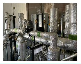
Corrosion under insulation (CUI) is a rampant problem in the oil and gas industry and other sectors where insulated piping is common. The same insulation that traps moisture also hides the resulting corrosion, meaning damage could be catastrophic before it is discovered. Cortec<sup>®</sup> offers a unique approach to fighting this problem through the application of Vapor phase Corrosion Inhibitors into existing insulation.
