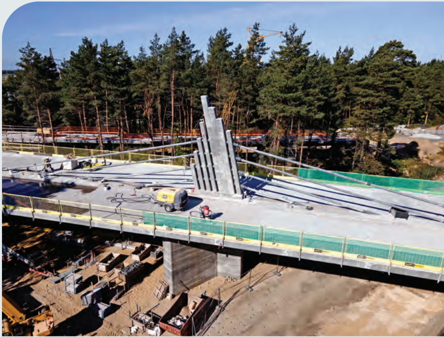
ABOVE: Figure 3 – Skulte overpass.
