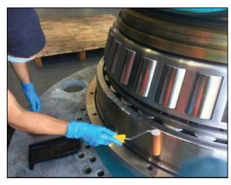
mils) wet film thickness using a roller. Finally, each element was wrapped and heat shrunk in either VpCI®-126 HP UV Shrink Film or MilCorr® VpCI® Shrink Film, depending on length of protection needed. The
