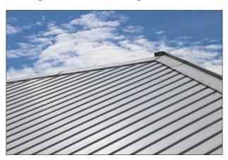
VpCI®-373 was used to answer the adhesion question when painting a galvanized roof over a liquid nitrogen loading dock at an industrial site in the Philippines. Lead and zinc chromate based primers had not been enough to avoid adhesion problems, and etching of the galvanized coating with phosphoric acid was expected to lead to coatings failure within a year. This time, the customer chose to clean the new roofing material and apply VpCI®-
