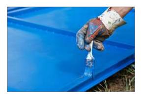
VpCI®-386 is a fast-drying water-based acrylic one-coat system topcoat that can be applied direct to metal for protection in harsh, outdoor, unsheltered applications. The complex mixture of corrosion inhibitors offers protection that competes with most paints and zinc-rich primers. VpCI®-386 has excellent UV resistance. It is also weldable and can be used to keep surfaces corrosion-free prior to welding. VpCI®-386 comes as a clear coat
