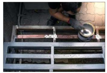
hardness of H in three to seven days. It provides high level 5B adhesion, integral to a good coatings bond.
