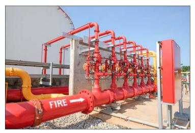
leaks or failures. Unfortunately, the damp environment created by hydrostatic testing could lead to corrosion and future leakage or clogging when the fire extinguishing system is actually needed. Including VpCI<sup>®</sup>-649 BD in hydrostatic test water can help systems avoid significant corrosion failures like these.
