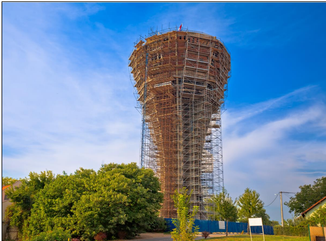
Vukovar Water Tower during the renovation phase.
