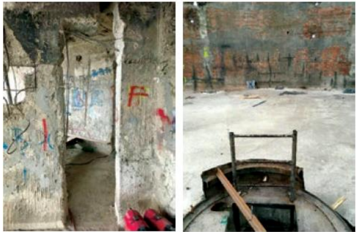
Vertical and horizontal surfaces before repair and impregnation.
