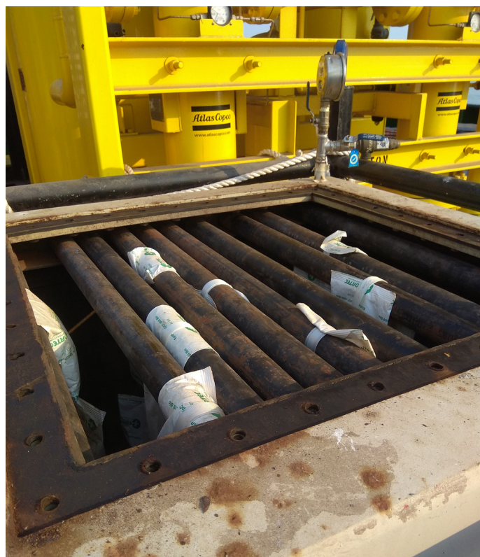
Figure 4. The VCI pouches were draped inside the plenum, and air was injected to carry the sublimated VCI vapors through the subsea pipelines. Image courtesy of Cortec Middle East.
