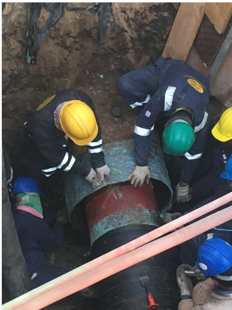
Figure 7. Preparing a cased pipeline crossing for VCI filler application. Image courtesy of Cortec Middle East.
