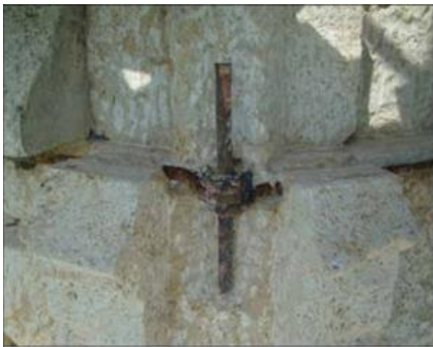
Left picture: Damaged steel bands. Right picture: CorrVerter® applied to the right side of the band; the coating has converted the corrosion into a protective layer.
