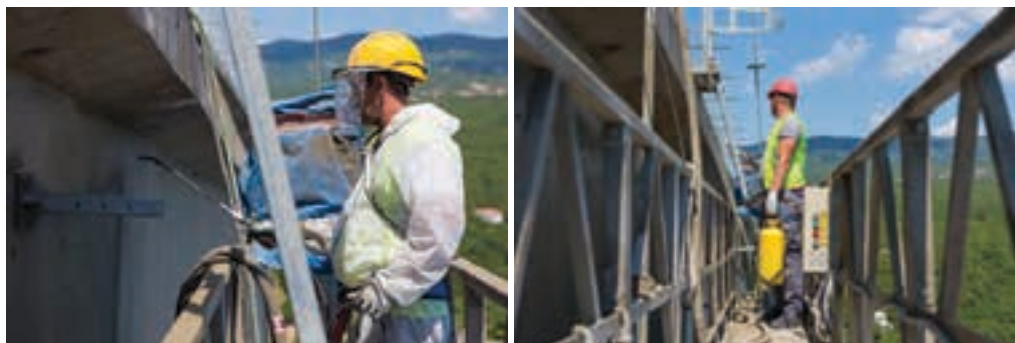
Application of MCI ® 2020 will stop further corrosion of reinforcing metals and extend the service life of the bridge.
