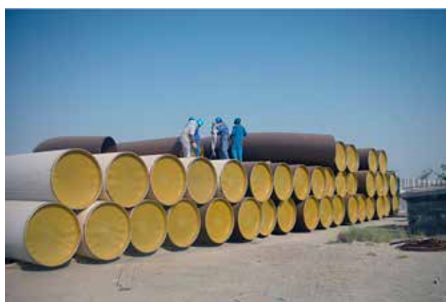
Figure 4. The opened end was sealed with an end cap. This would ensure the protection of the pipes for more than three years.
