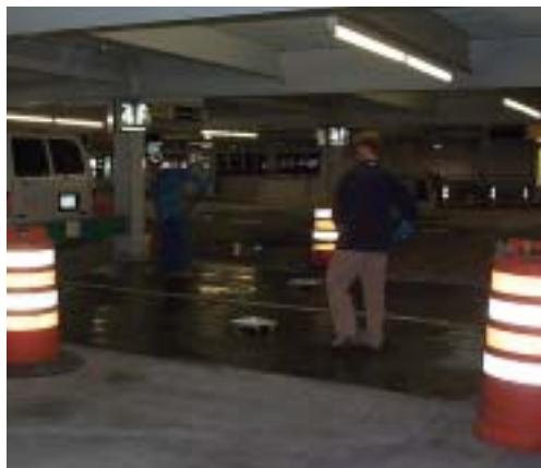
MCI 2020 has been included in a test on a parking ramp at La Guardia Airport in New York.
