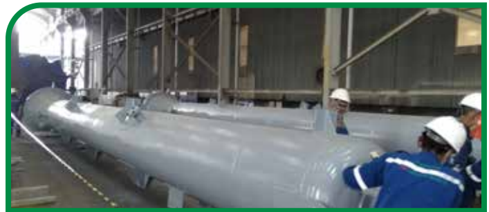
PROTECTING NEWLY FABRICATED EQUIPMENT Case History #698
