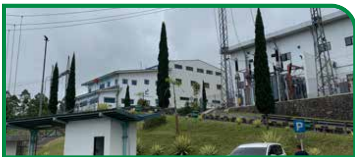
PROTECTING ELECTRICALS/INSTRUMENTATION AT GEOTHERMAL POWER PLANT Case History #712
