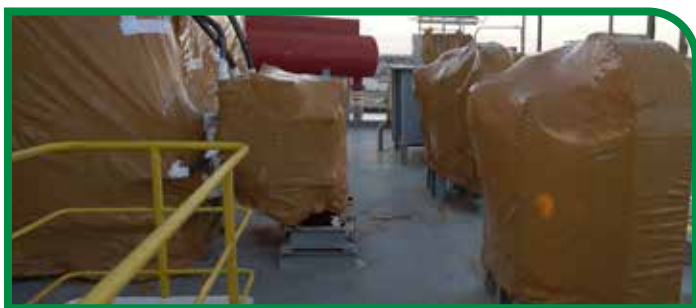
PRESERVATION OF OFFSHORE RIG TO WITHSTAND HURRICANE HARVEY Case History #662
