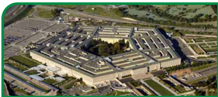
RESTORATION OF PENTAGON LIGHTWELL WALLS Case History #46
